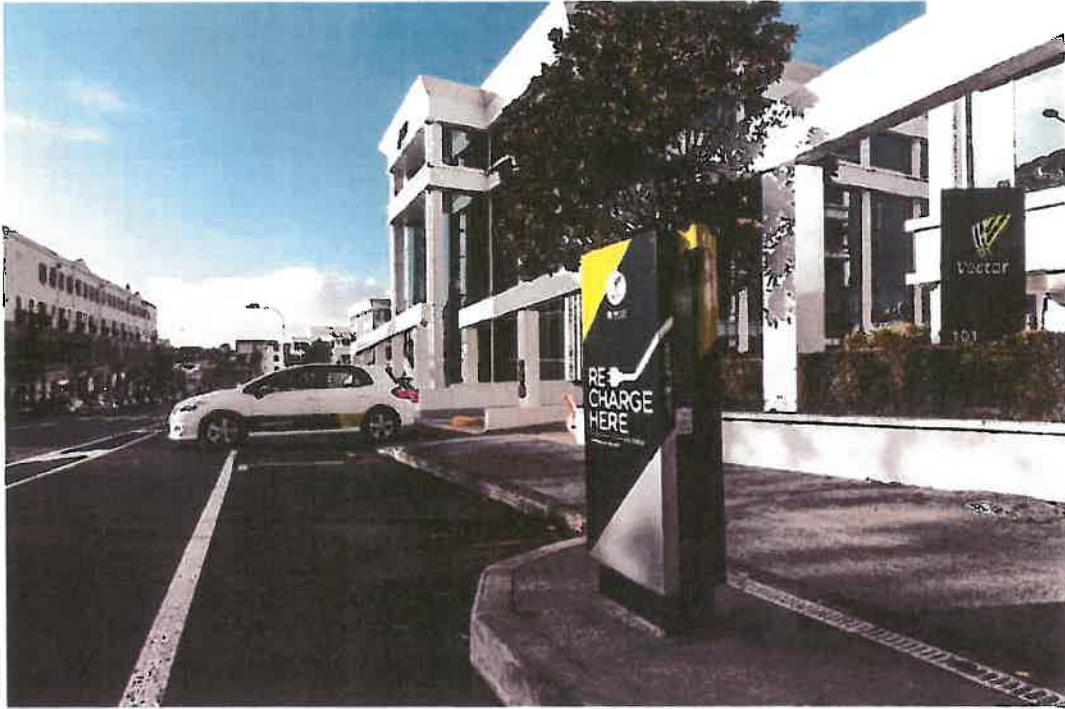
Electric Vehicle charger station installation at 101 Carlton Gore Road
