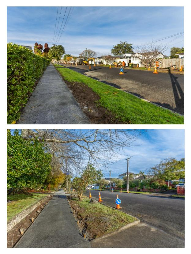
These images are of progress on the large scale Mt Albert Undergrounding Project. The photos show new footpaths that have been reinstated over top of the new underground electricity networks laid in the street. Houses are being systematically connected to these new underground cables, and when they are all connected the old overhead lines and poles will be decommissioned and removed.
