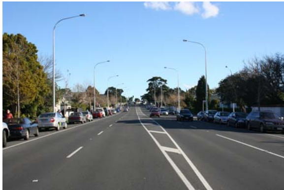
Jervois Road after
